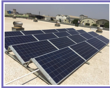
Solar Panel Structure Mounting on RCC
