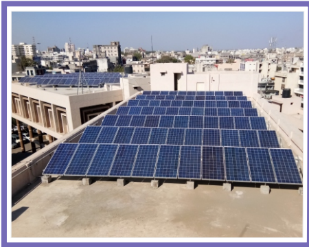
Solar Panel Structure Mounting on RCC
