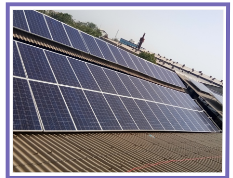
Mounting on Cement Roof
